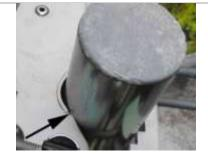
Set the elevation of the dish to the figure that was calculated for you using the Ka-Sat dishpointer tool in step 1. Make sure that the elevation fixing bolts are loose and turn the elevation adjustment bolt until the correct angle is reached. Note where you measure the angle in the picture ... this one is set to nearly 36°
